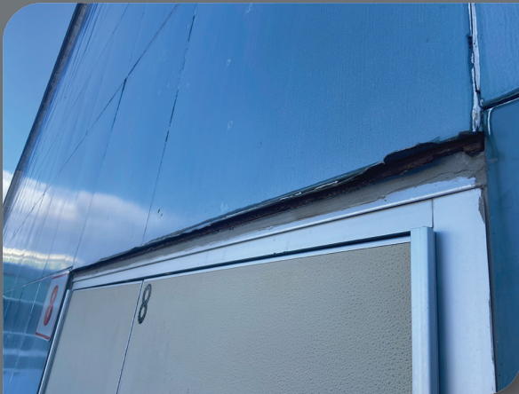
Rust, warping and sealant gaps evident in the tile on the exterior wall of the auditorium.
