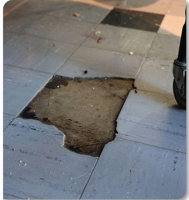
BELOW The Glenclyff Elementary School cafeteria floor has multiple tiles that are chipped and missing. This project includes elementary cafeteria renovations such as new flooring and lighting systems.
