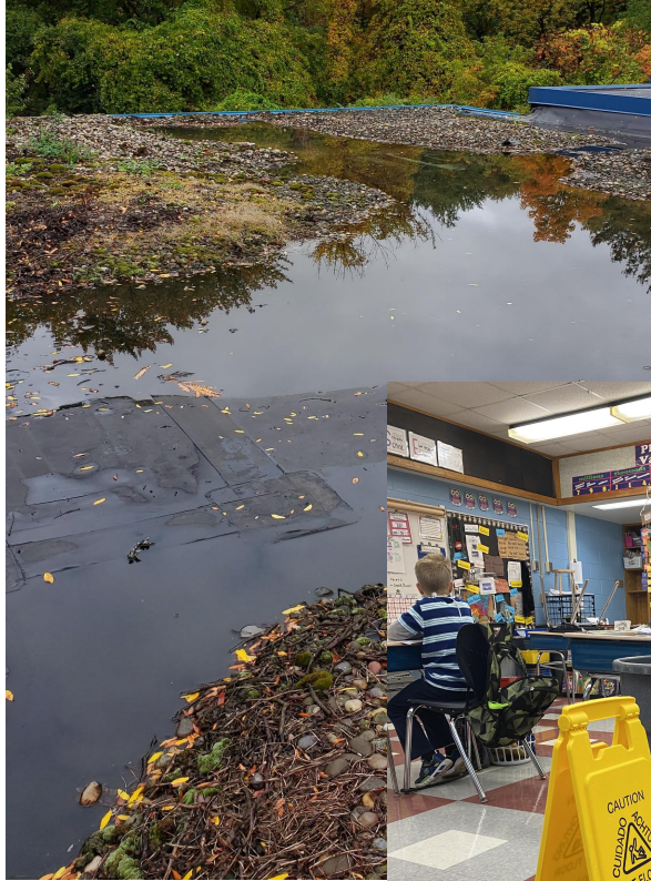
Glencliff Roof: Pooling Leaking into Classrooms
